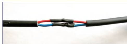
2. Seal the cable with the shrinkable tube.
